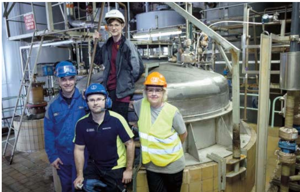
Iggesund's Hans Nilsson (left) and Morgan Arousell, process operator, at the retrofitted chlorine dioxide plant. Photo also includes Kimona Häggström and Helena Falgén with AkzoNobel.
