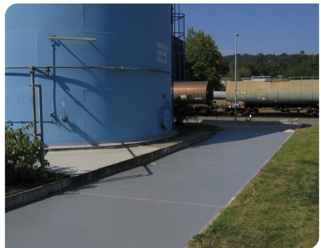
Picture 3: Polysulfide based joint sealant as a crack-bridging, chemically resistant coating
