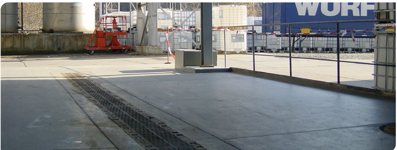
Picture 4: Floor coating of a truck-wash station in a chemical plant
