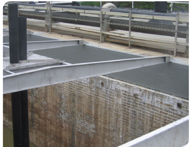
Picture 6: Thioplast® EPS polysulfide coatings of sewage plant
