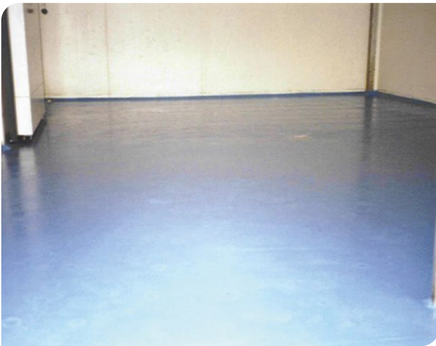
Picture 2: Thioplast® EPS polysulfide coating of the floor in a slaughterhouse
