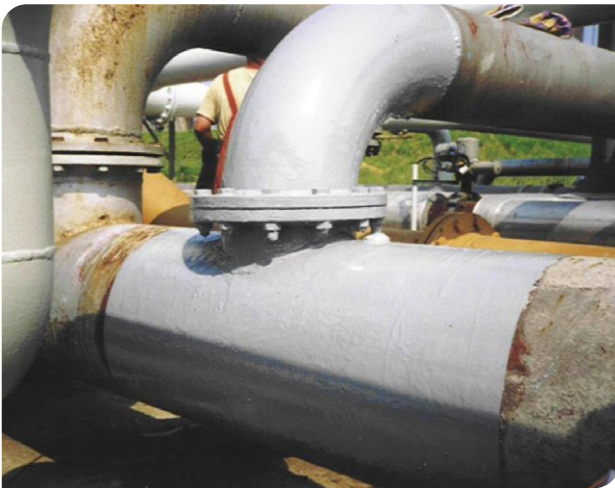
Picture 5: Heavy-duty corrosion protection of industrial shipping
