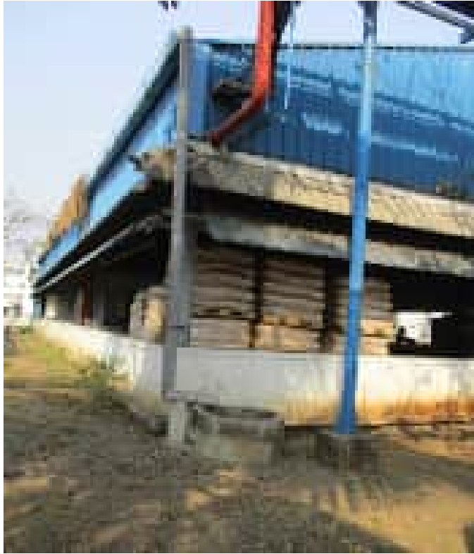
1. Rainwater recharge pit of Warehouse roof
